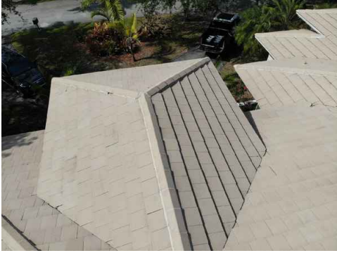
Photos of Each Slope
